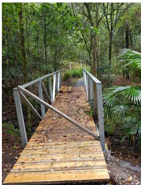
Decking for approaches completed Fern Gully bridge. Photo: Marie Mathews Repairing road damage from March 2022 Rain Event. Photo: Tracey Whitby
