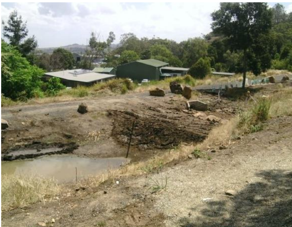
Figure 2: The pond in the Sensory Garden being built with a weir to divide the deep end from the overflow area, Nov 2014
